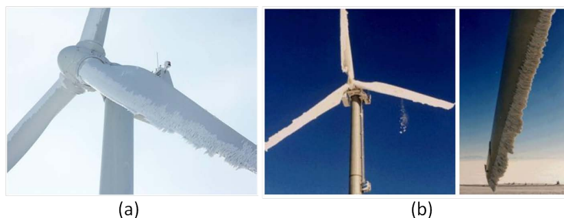
Figure 1.3: (a) Ice accumulation on the leading edge of wind turbine blades causes reduced turbine availability, and if operated, potentially damaging loading and increased public safety concerns. Photo by: Kent Larsson, ABvee (SE) from Ref. [5]; permission received from Goran Ronsten; (b) Ice accumulation may either fall off or be thrown off, causing safety issues for persons, animals, or properties that may be nearby. Photos are of 150 KW Grenchenberg turbines in Switzerland; photograph from Ref. [25]; permission received from Robert Horbaty.
